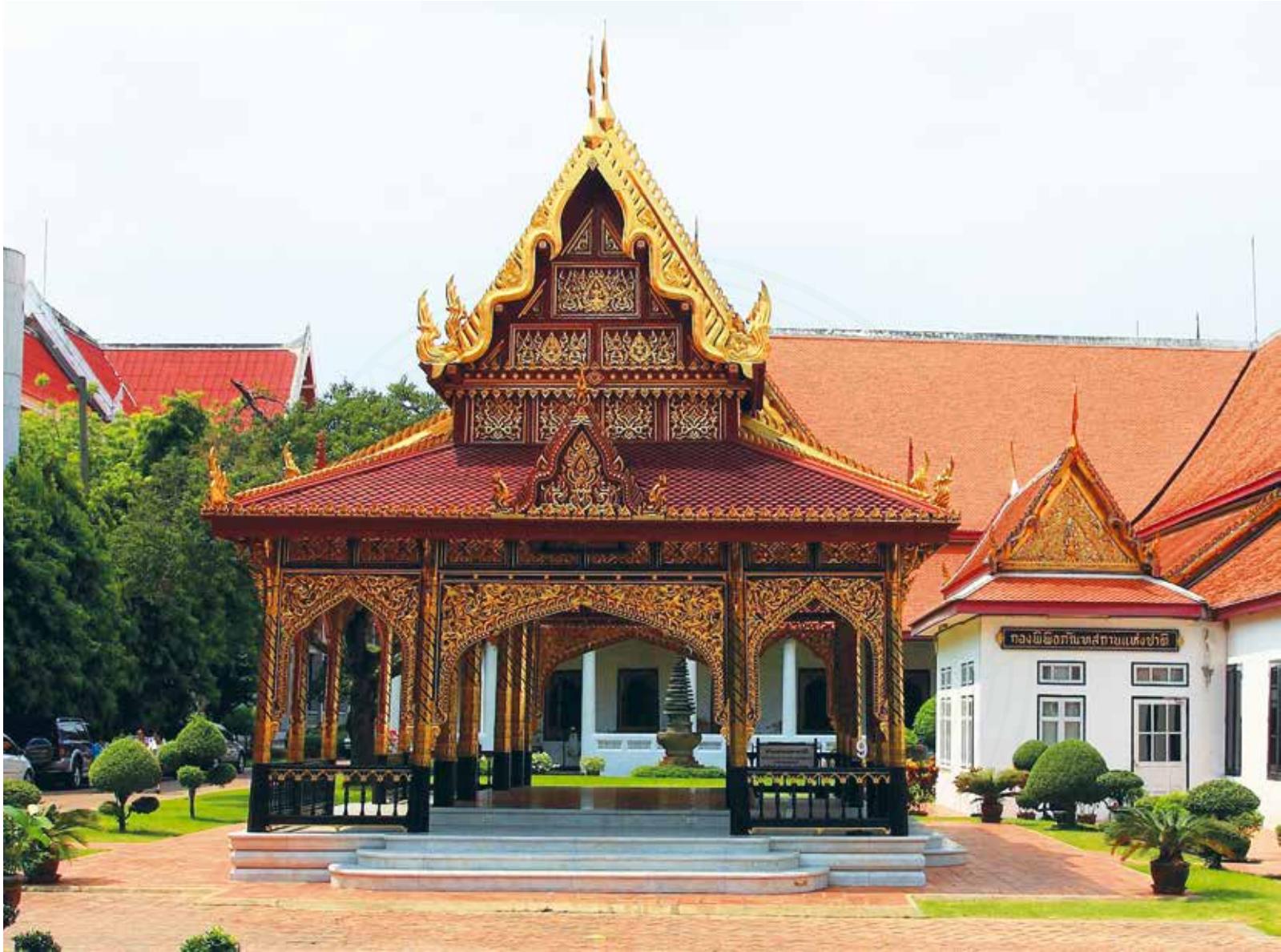
Sala Samran Mukkhamat, a typical Thai Sala, Palace to the Front, Bangkok.
