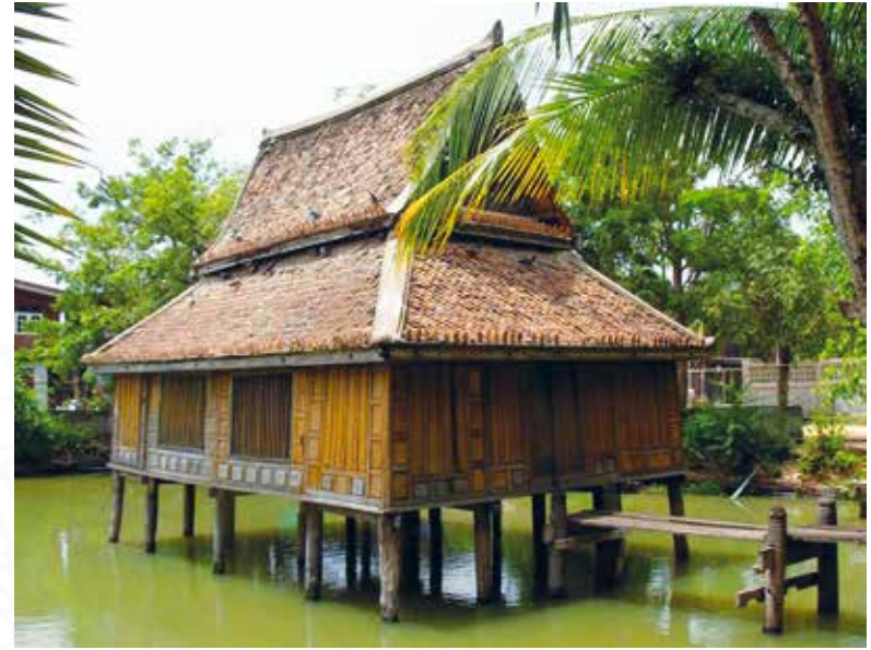
Ho Trai, Wat NaPhra That (Wat Ta Khu), PakThong Chai, Nakhon Ratchasima. To prevent the white ants harming the holy-book of palm-leaves the libraries were erected over ponds of water.
