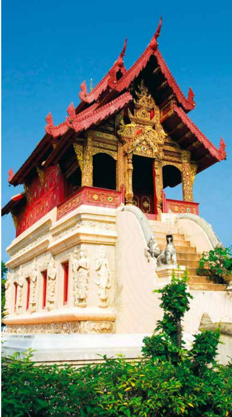
Ho Trai, Wat Phra Sing, Chiang Mai, build by King Kavila in 1811 Some of the northern Thai Ho Trai have the ground floor built of bricks and the upper floor of wood.
